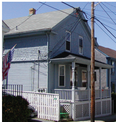
THE C.W. AND N.E. NORTH HOUSE
