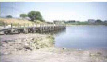
Galilee at Great Island Bridge
