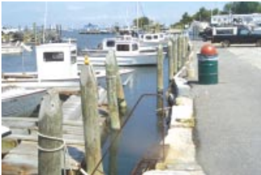
Wickford Municipal Wharf
