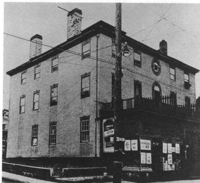
Fig. 16: Samuel Whitehome House (1811), 414-418 Thames Street, before renovation.
