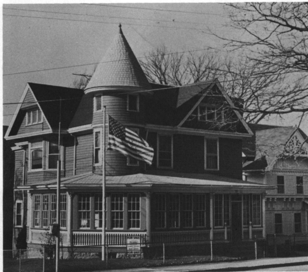
Fig. 48: J. B. Parsonage House (c. 1900), 525 Spring Street.
