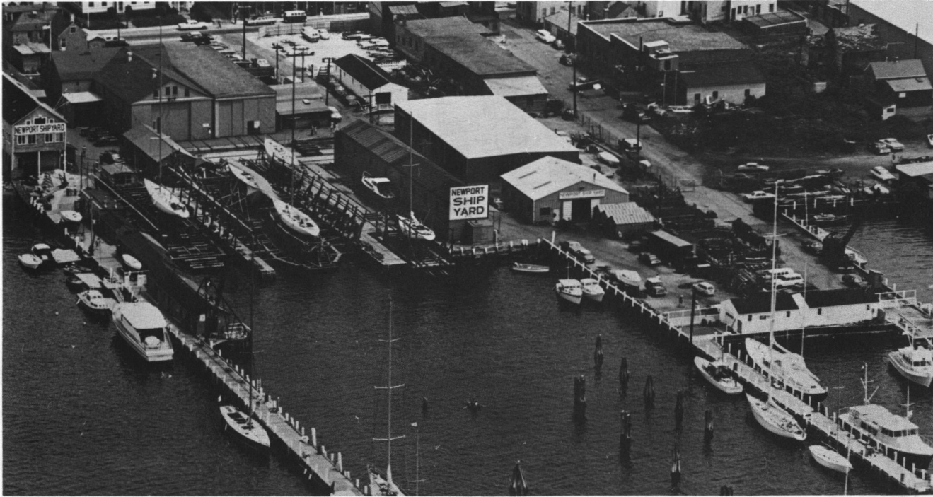
Fig. 25: Newport Shipyard, now Newport Offshore Ltd. This property has been a shipyard since 1834 when it was purchased by Silas Cottrell. In the mid-18th century merchant Josiah Brown's wharf was located here.
