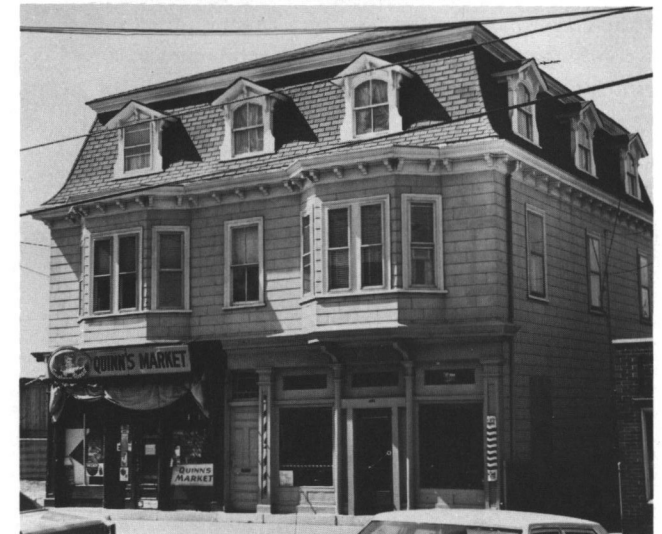
Fig. 31: J. J. Lynch Building (1886), 491-495 Thames Street.
