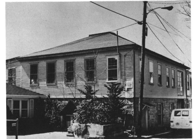
Fig. 58: 16 Coddington Wharf (the last surviving portion of the Coddington Mill complex) before renovation.
