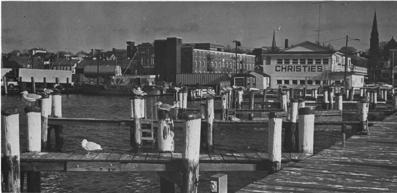
Fig. 26: View from Hammett's Wharf, showing (from left to right) the Perry Mill as it exists today, Christie's Restaurant and St. Mary's Church.
