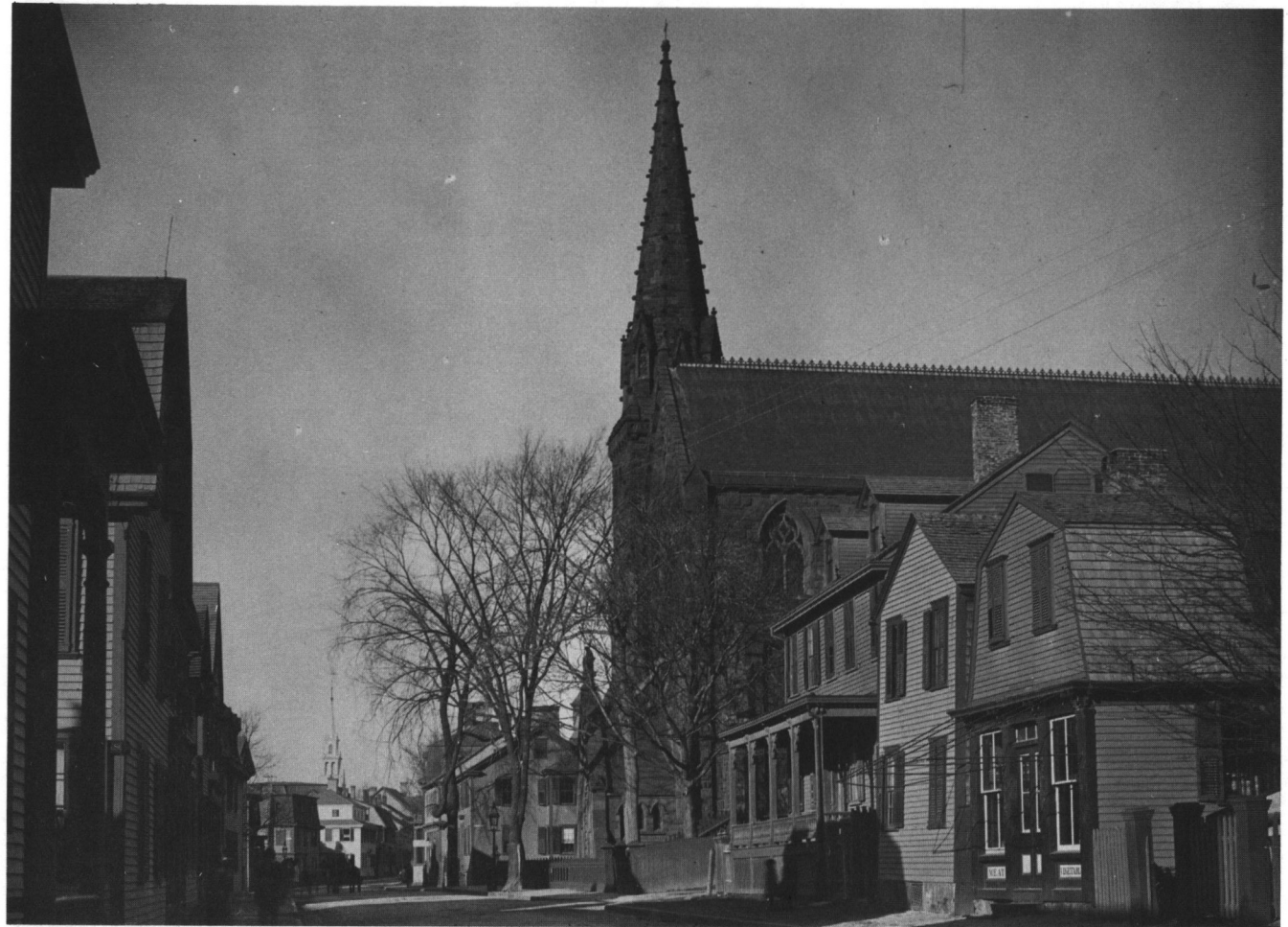
Fig. 36: View north up Spring Street in about 1875; St. Mary's Church is on the right and the steeple of Trinity Church is in the background.
