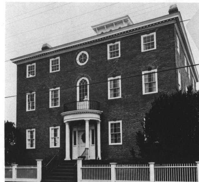
Fig. 17: Samuel Whitehome House (1811), 414-418 Thames Street, after renovation.
