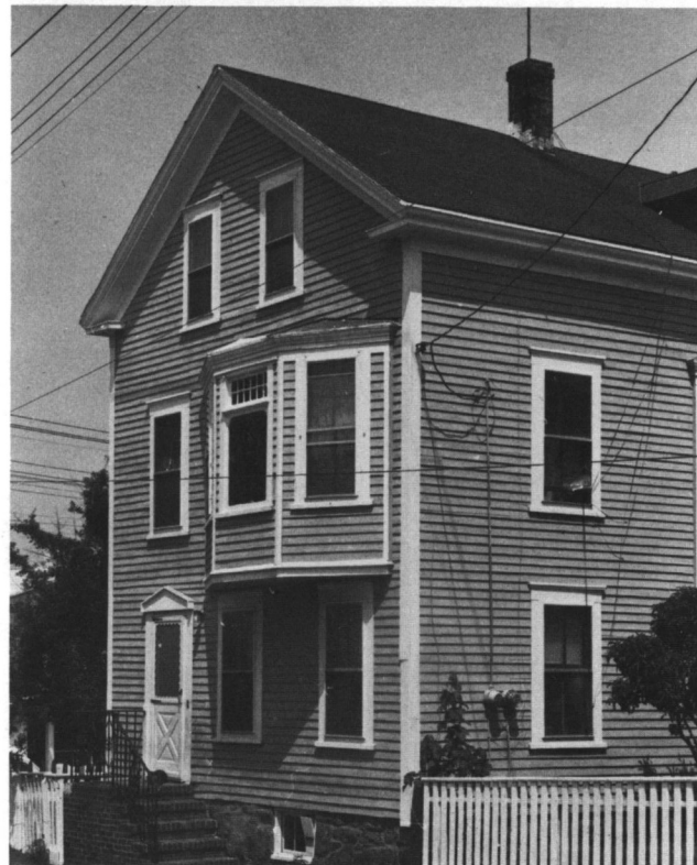
Fig. 55: John France House (c. 1860; altered c. 1890), 8-10 Howard Street.
