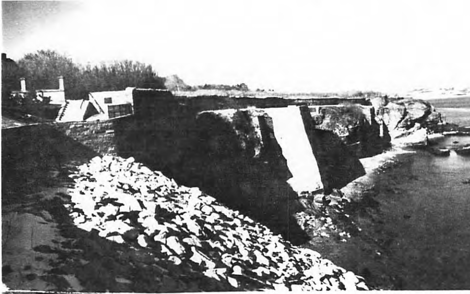
Most recent construction - Webster Street.
